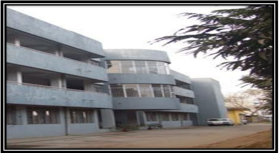
Multi-Storied Hostel Building for IIE at Guwahati
